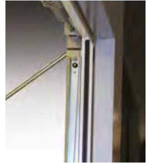
Anti drop mechanism. Large spindle roller. Spindle roller bracket has a reinforcement bracket to stop excessive movement.
