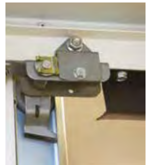
Anti drop mechanism. Large spindle roller. Spindle roller bracket has a reinforcement bracket to stop excessive movement.
